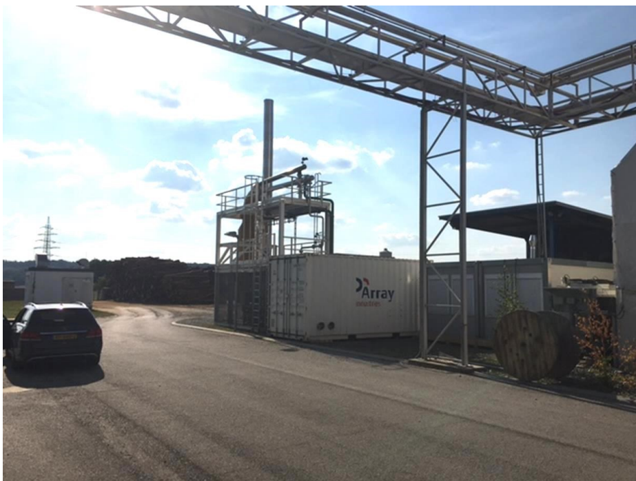
Pilot installation in Güssing (Austria)
