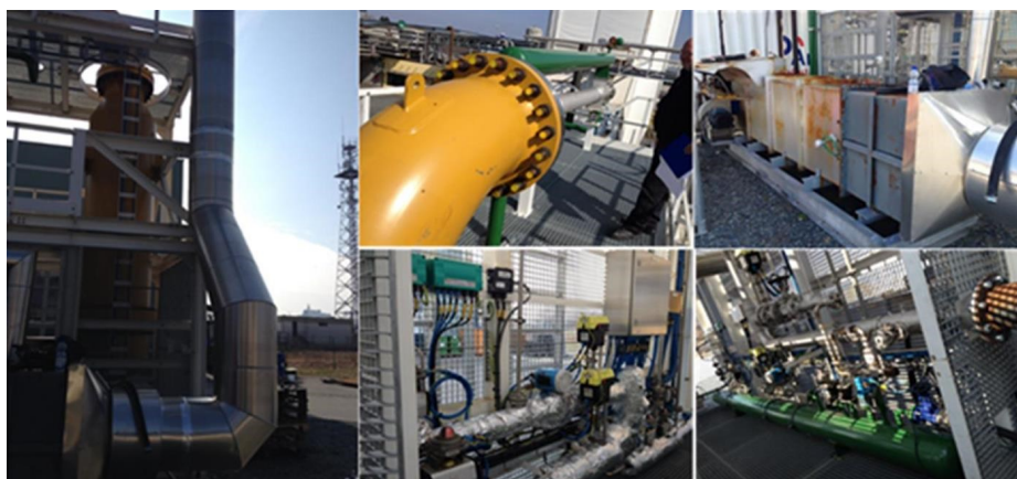
Pilot installation in Güssing (Austria)
